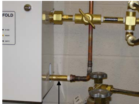
Intermediate relief valve connection 1/2" NPT brass nipple provided shown)
