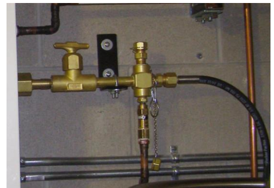
20" header length (Header pictured above accommodates 2 - 72" flexible pigtails for 2 portable bulk vessels, plus relief valve with pipe away)
