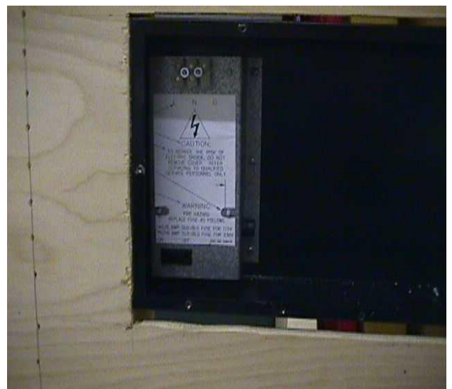
Figure 13 – Install Power Supply
